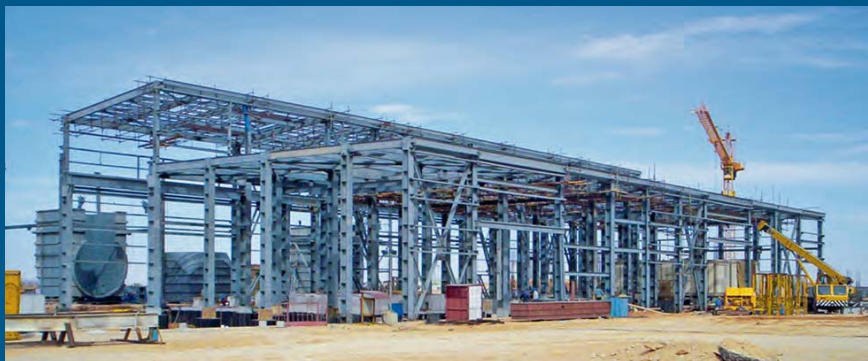
Structural steel work for Rouis power plant
